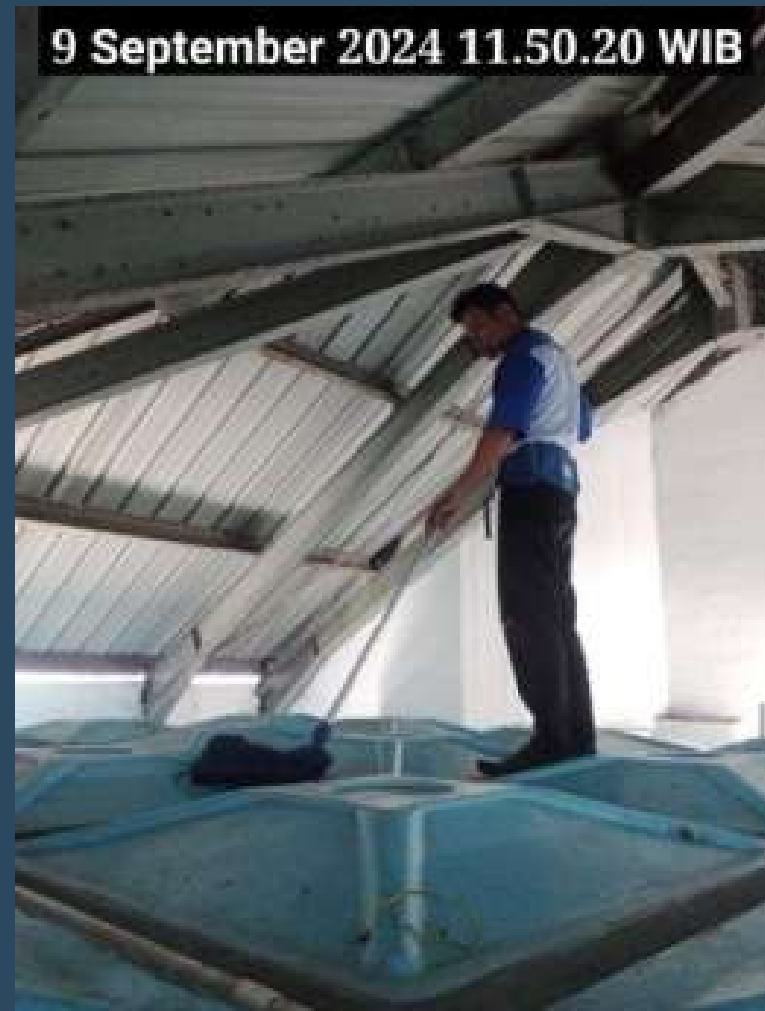
PEMBERSIHAN WATER TANK ROOF TOP ALL TOWER
